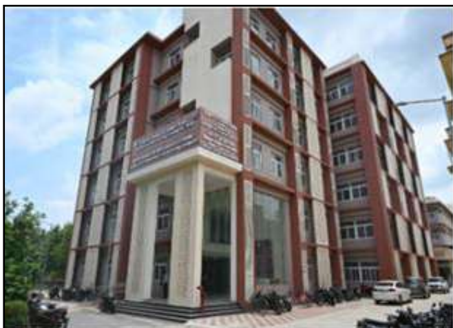
Photo-1 : Front View
